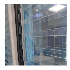
Polycarbonate Bars provide attractive, transparent window protection and are ideal for offices that don't require highly visible burglar proofing.
